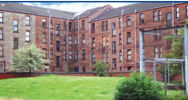
Rathlin Street - site for new-build development
