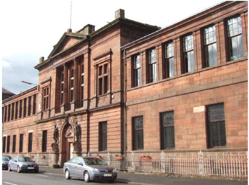
Fairfield following restoration of windows
